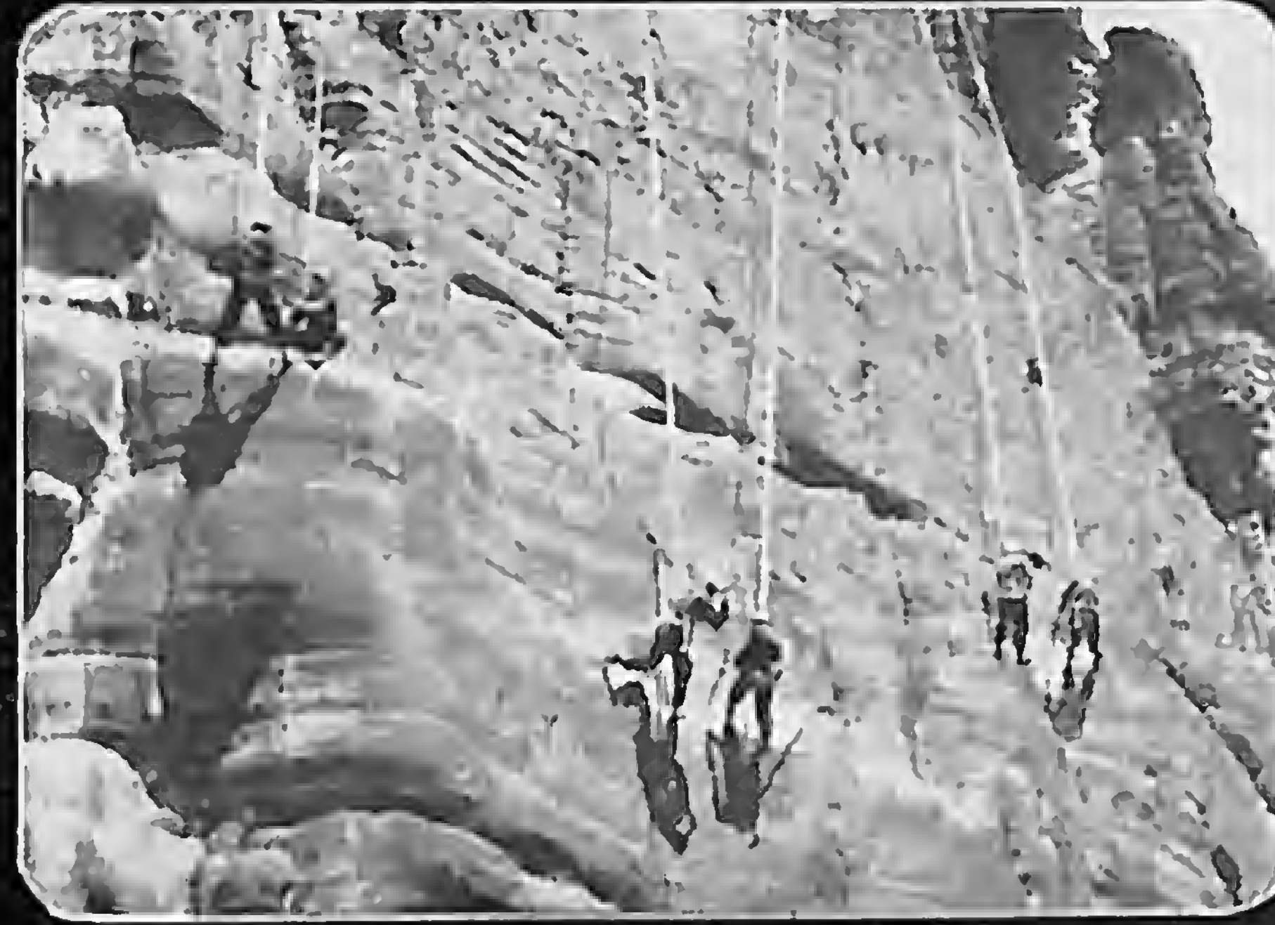
The canal will cross this cliff.
